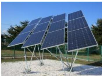
(f) Photograph of 0.940 m × 1.56 m bifacial modules of 12 sets, orientation of 0°
