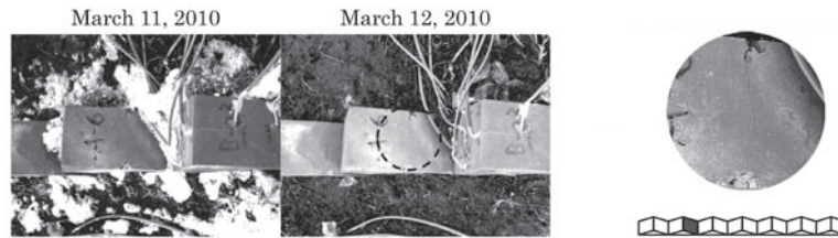
Fig.26 Crack of the brick No.2 that occurred at (a) Snow removal (Picture taken on March 11 & 12, 2010) .
