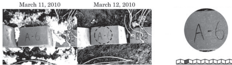
Fig.25 Crack of the brick No.2 that occurred at (a) Snow removal (Picture taken on March 11 & 12, 2010) .
