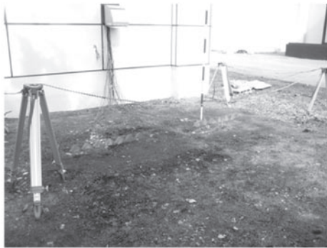
Fig.15 Appearance of exposure experiment site (Picture taken in April, 2009).
