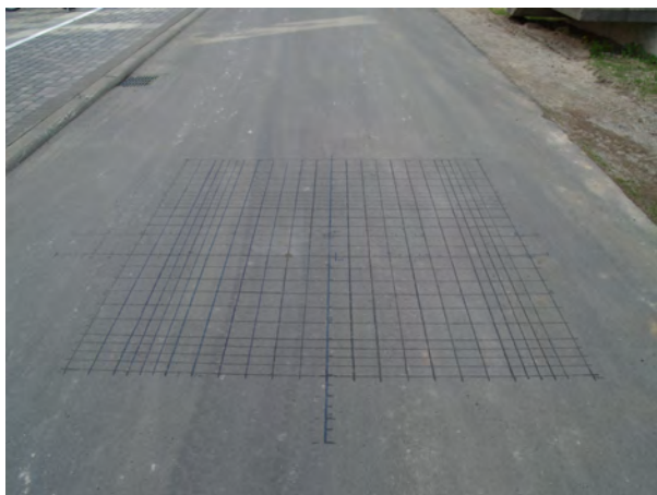
Fig.3 Measurement grid on asphalt road.
