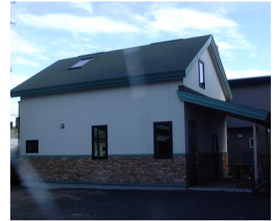
(a) Schematic (b) Exterior view Fig. 1 Renewable energy system with a GHP-powered floor heating
