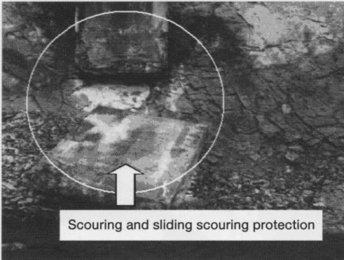
Photo.2.3 Scouring part of A1 of Dairokuotofukegawa Bridge
