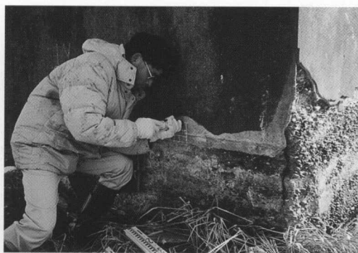
Photo. 4 Schmidt hammer test on face of external wall
