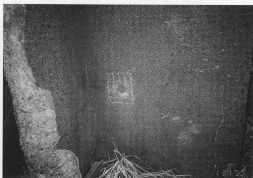
Photo. 8 A spot at Schmidt hammer and sampling
