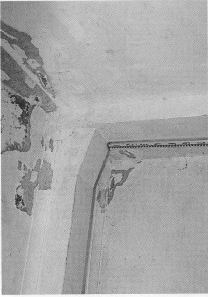
Photo. 21 Solid wall girder, ceiling girder and a partition wall between main room and cable-pit room at the center of the interior comparatively one-storied building, as measure fore earthquake proofing
