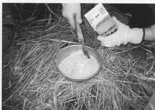
Photo. 6 Repair material for drilled hole
