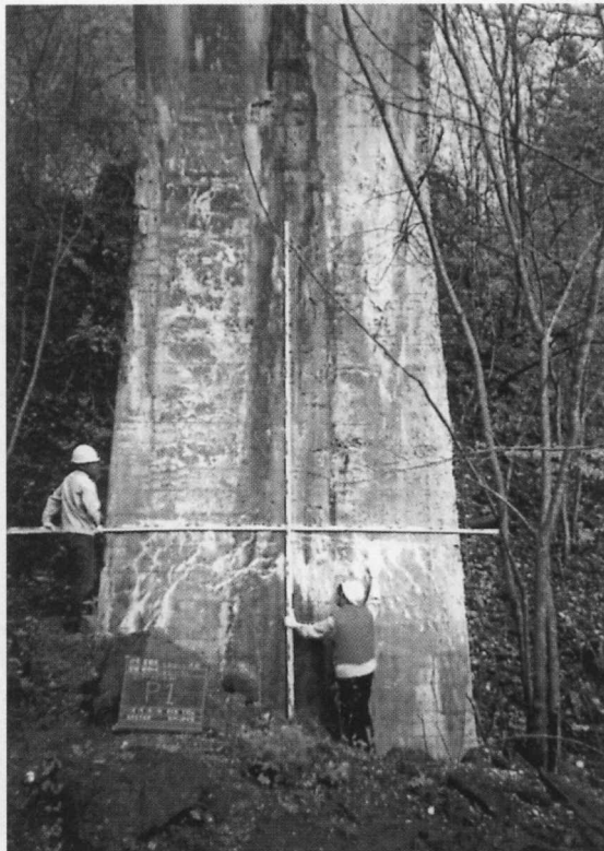
Photo. 5 The surface of bridge pier (1P from Obihiro side) for non-destructive test of Dai San Otofuke Bridge
