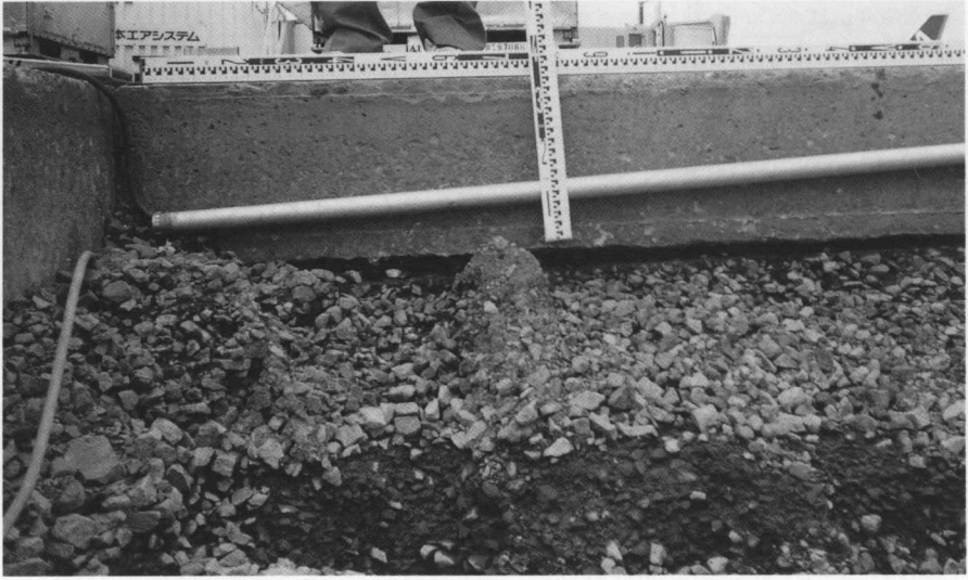
Photo-1 Old concrete plate of the airport apron.
