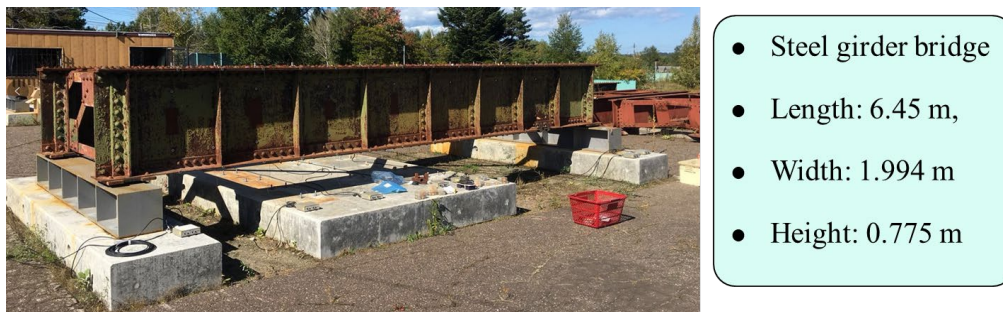
Fig. 1. Basic information of the bridge
