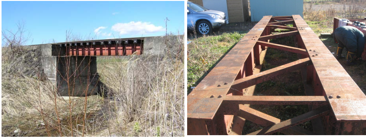
Photo 1 Railway Bridge photo used for measurement (Assembled steel I beam, length 6.96m Railway bridge)
