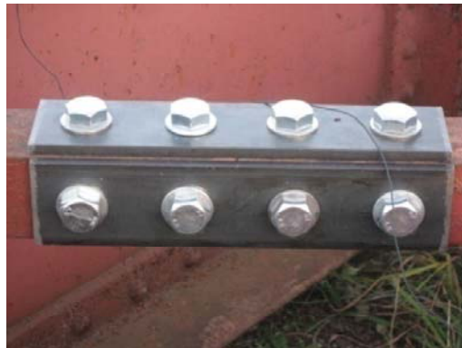
Photo 4 Splice connection of lateral member by bolts ( D0 )
